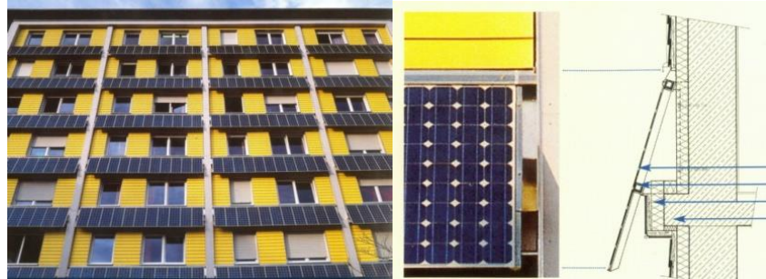
Figure 5. Integration of photovoltaic modules in the façade of the Catholic Apprentice Dormitory, Germany, http://www.pvdatabase.org/projects_view_detailsmore.php?ID=265
