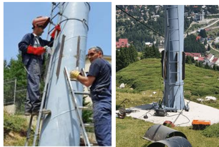
Figure 12. Welding temporary ribs
