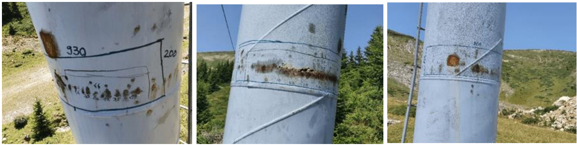
Figure 11. Columns for repairing
