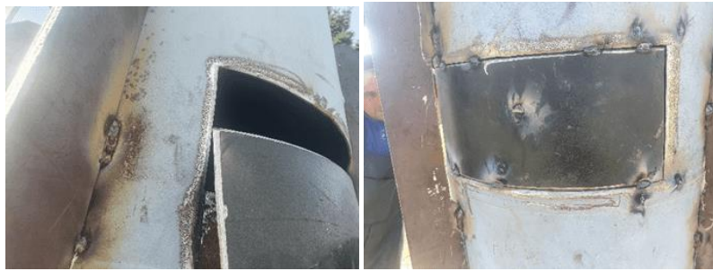
Figure 15. Tack welding
