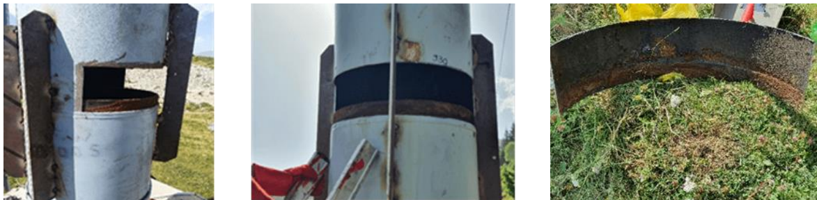
Figure 13. Columns after cutting
