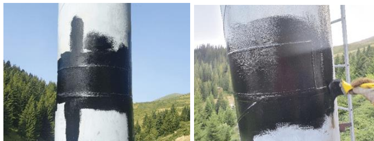
Figure 17. Painting of welded segments
