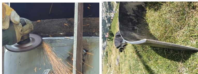
Figure 14. Preparing of parts for welding
