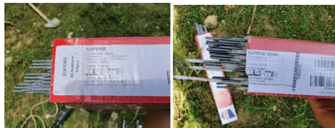
Figure 9. Electrodes used for repairing columns according to prescribed technology
