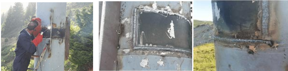
Figure 16. Welding of embedded segments
