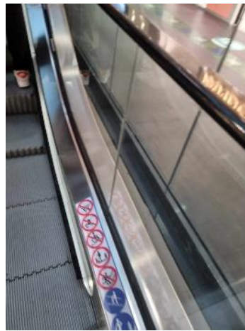
Fig. 15: Glass as a railing in an escalator in East Gate Mall – Skopje. Source: the author.
