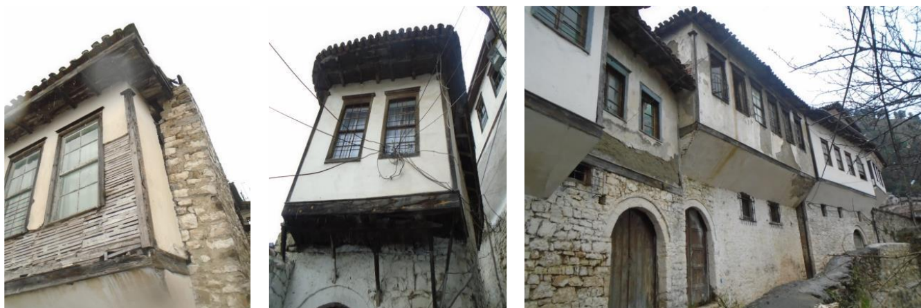
Figure 18. The construction of walls with a bondruk system (a), stone used for the construction of the first level, and wood for the other following floors (b) and (c). (source: authors)
