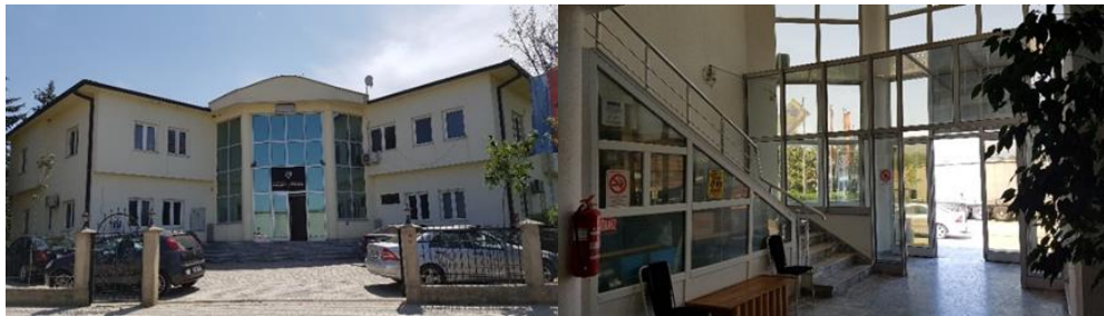
Figure 1: The building of the RLA building of the Municipality of Želino: a) north facade, b) entrance hall
