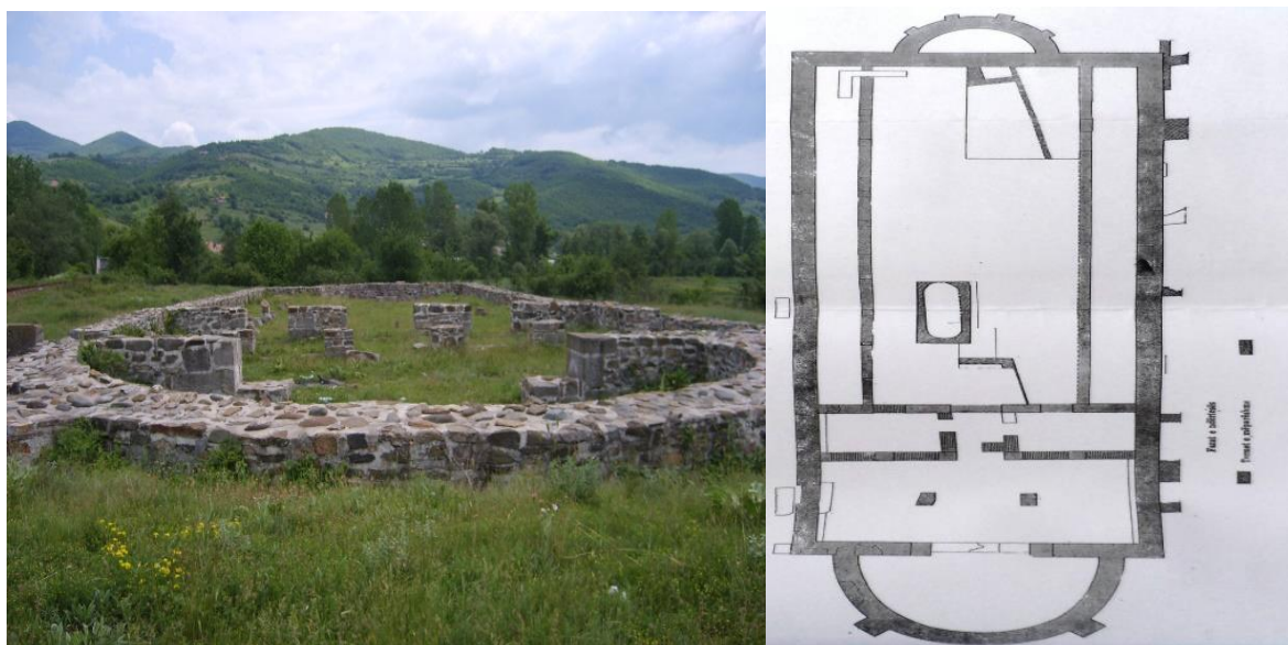
Fig. 5. 6. Basilica in the DD Municipality, as well as the plan of the basilica
