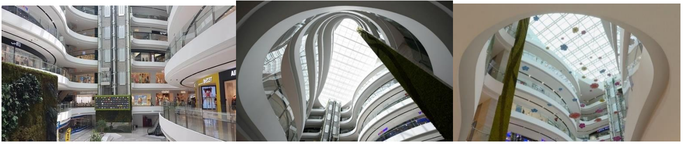
Figure 31. (a)(b)(c). View of the parabolic shapes inside the structure
