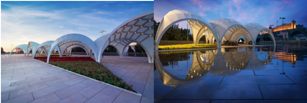
Figure 24. (a)(b) Hyperbolic construction on Skenderbeg Square
