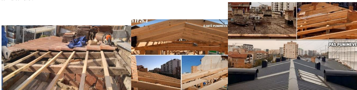
Figure 5. The existing state and after the renovation of the roof
