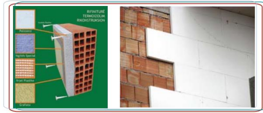
Figure3. Insulation of external walls
