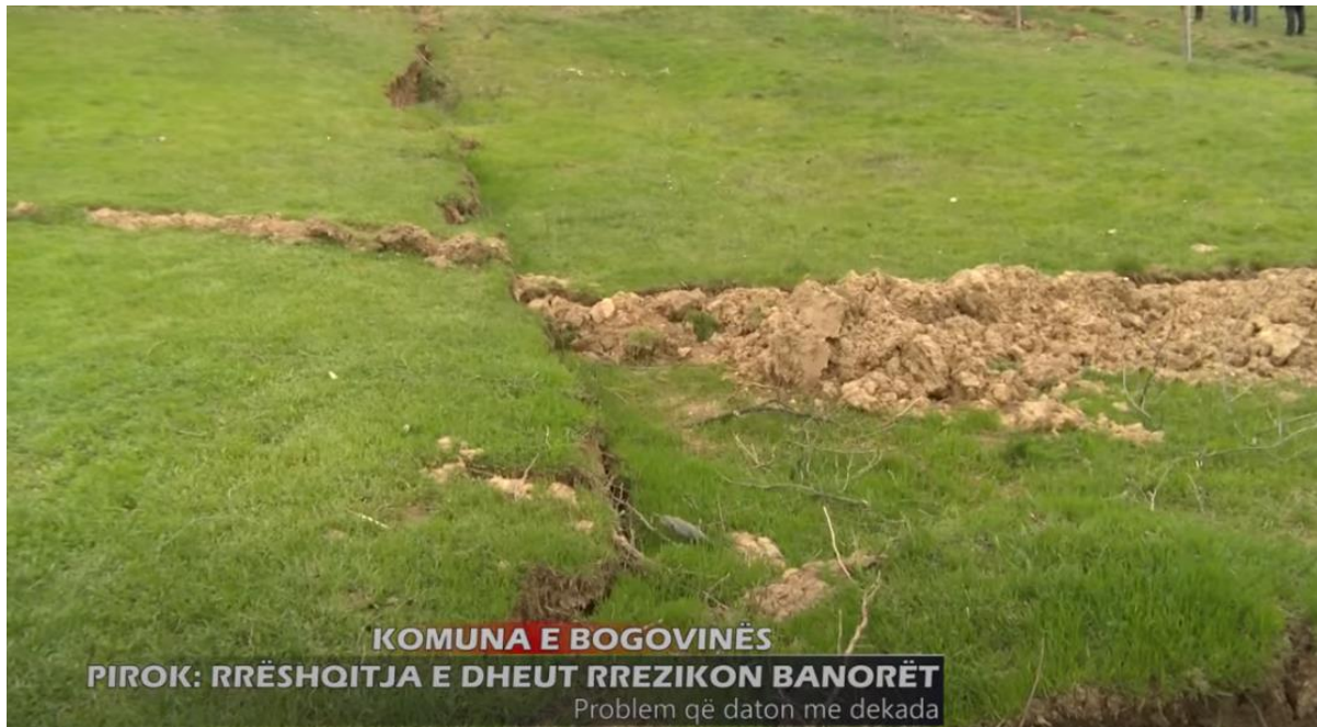
Figure 2. Landslide in the investigated locality
