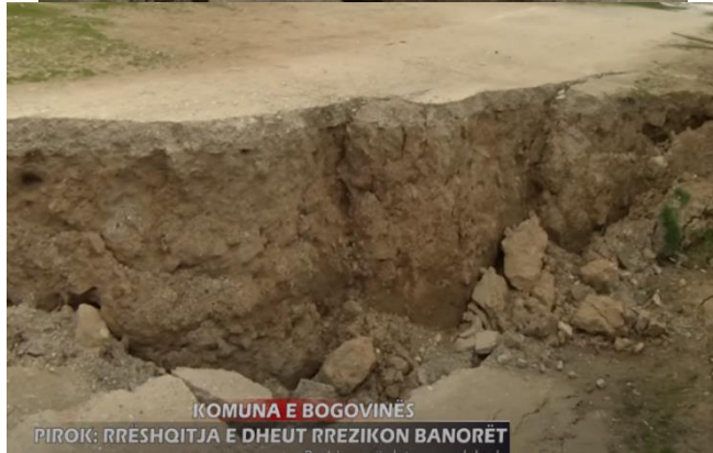
Figure 1. The appearance of cracks and landslides
