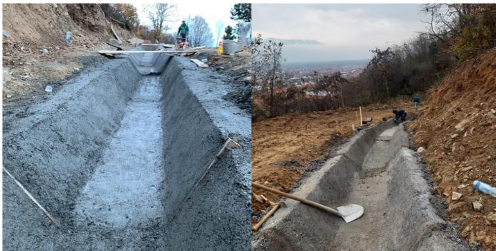
Figure 6. Channels for removing surface water
