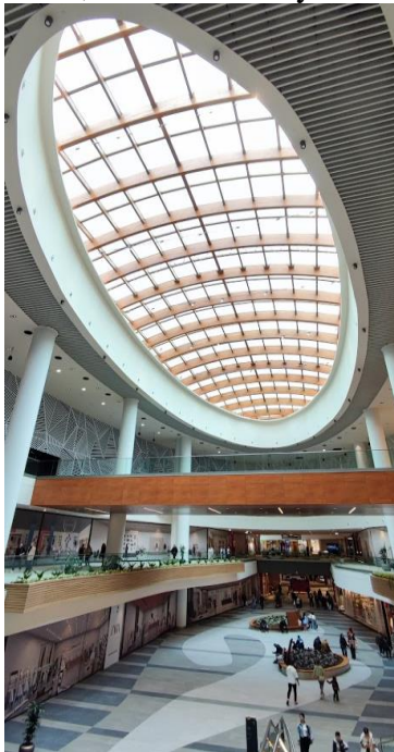
Figure 2.2.1 Quadrilateral mesh in Prishtina Mall (2022), Kosova
