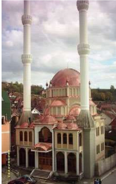
Figure 1. Çarshi Mosque in Rahovec
