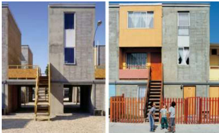
Figure 4. Home before and after extension by residents, Quinta Monroy, Iquique, Chile (courtesy of The Guardian)
