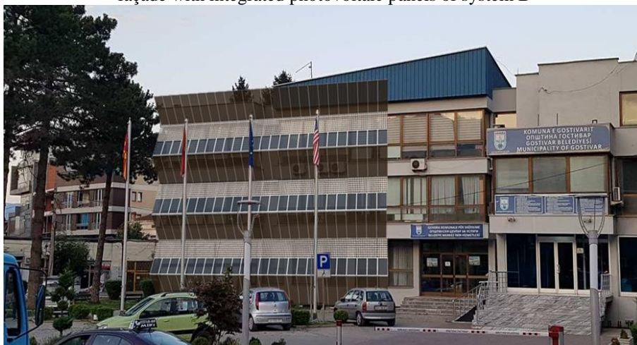
Figure 6. Appearance of the western façade of the Gostivar Regional and Local Government Building: partially clad double façade with integrated photovoltaic panels of system C
