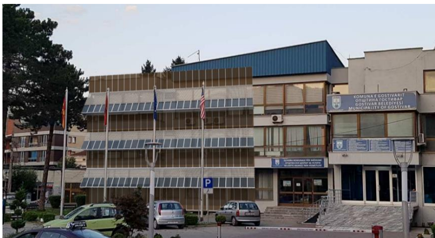
Figure 7. Appearance of the western façade of the Gostivar Regional and Local Government Building: partially clad double façade with integrated photovoltaic panels of system D
