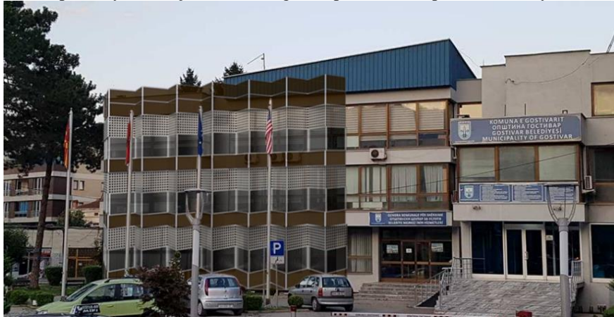
Figure 5. Appearance of the western façade of the Gostivar Regional and Local Government Building: partially clad double façade with integrated photovoltaic panels of system B
